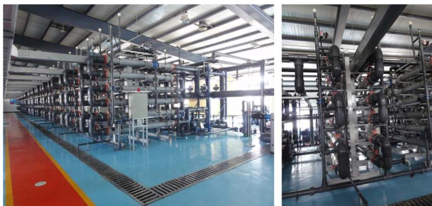
Fig. 1. Images of the pilot-scale UF set-up (with a treatment capacity of 9800 t per day).
