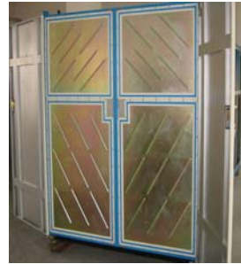
图 2 机柜门用钢板密闭 Fig.2 The cabinet door sealed with steel
